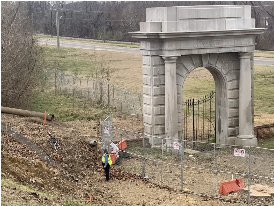
Adela and Jasper working the lower portion of the landslide area.
