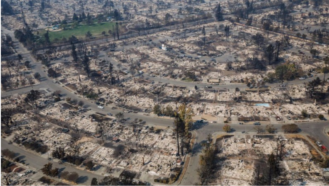
Fire damage in one Santa Rosa neighborhood.
